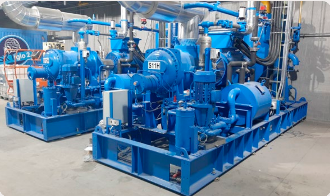
Capturing the residual heat from the cooling oil in our compressors to generate warm water for cleaning purposes
