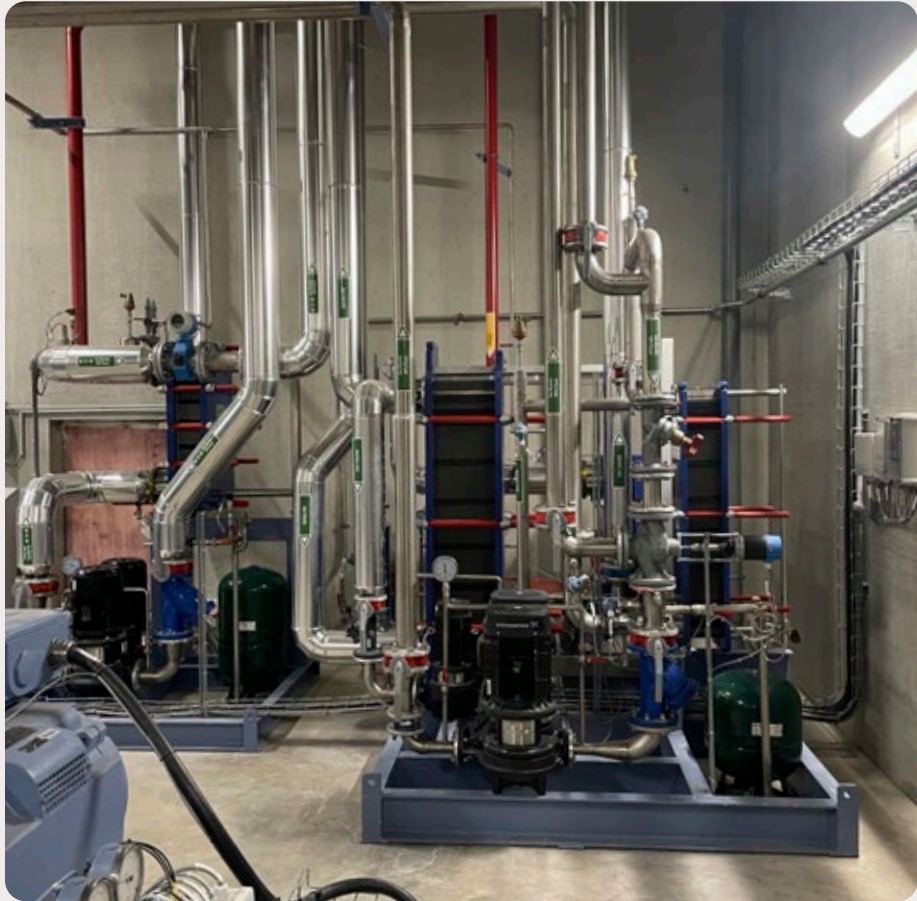
Heat recuperation at our site in La Garde-Adhémar
