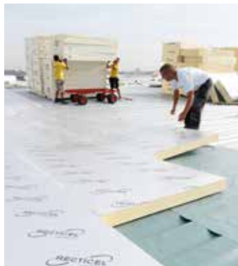
Roof insulation (flat and pitched roofs)
