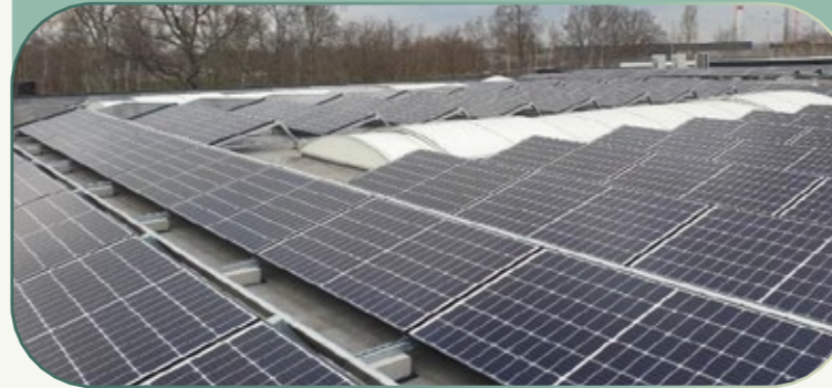
INSTALLATION OF SOLAR PANELS
