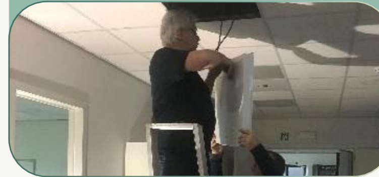
INSTALLATION OF LED LIGHTING
